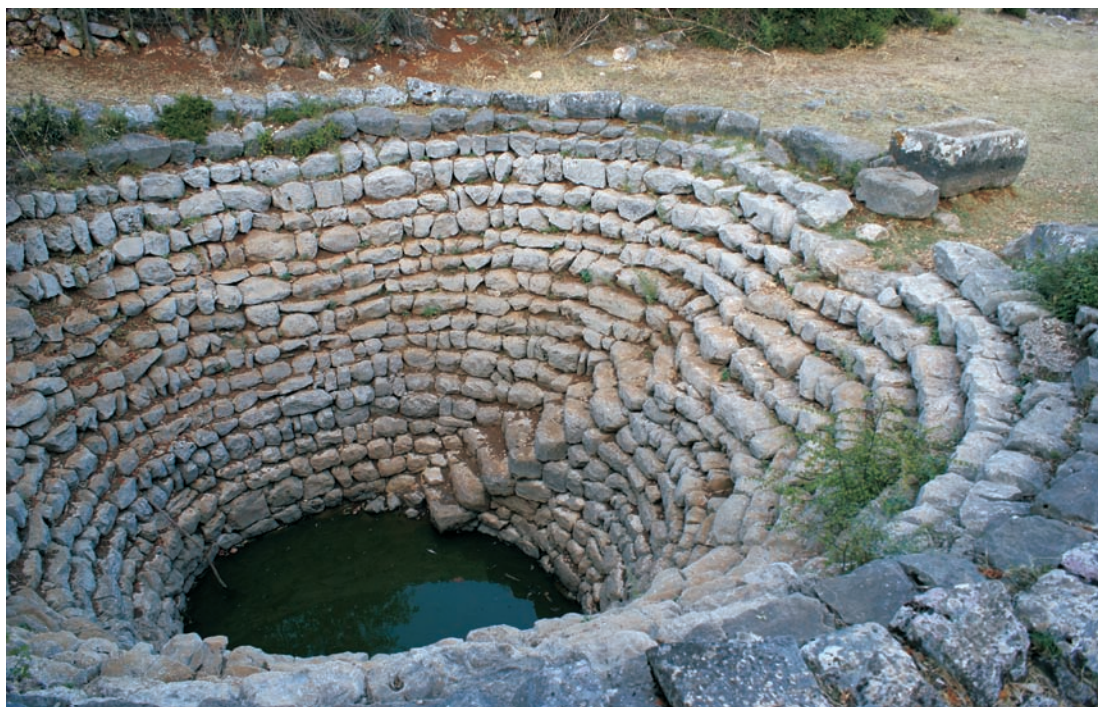
Fig. 35: Water reservoir built in the bottom of small doline in Boljuni, near Stolac in Herzegovina. This water was used for animals only (photo: A. Mihevc).
